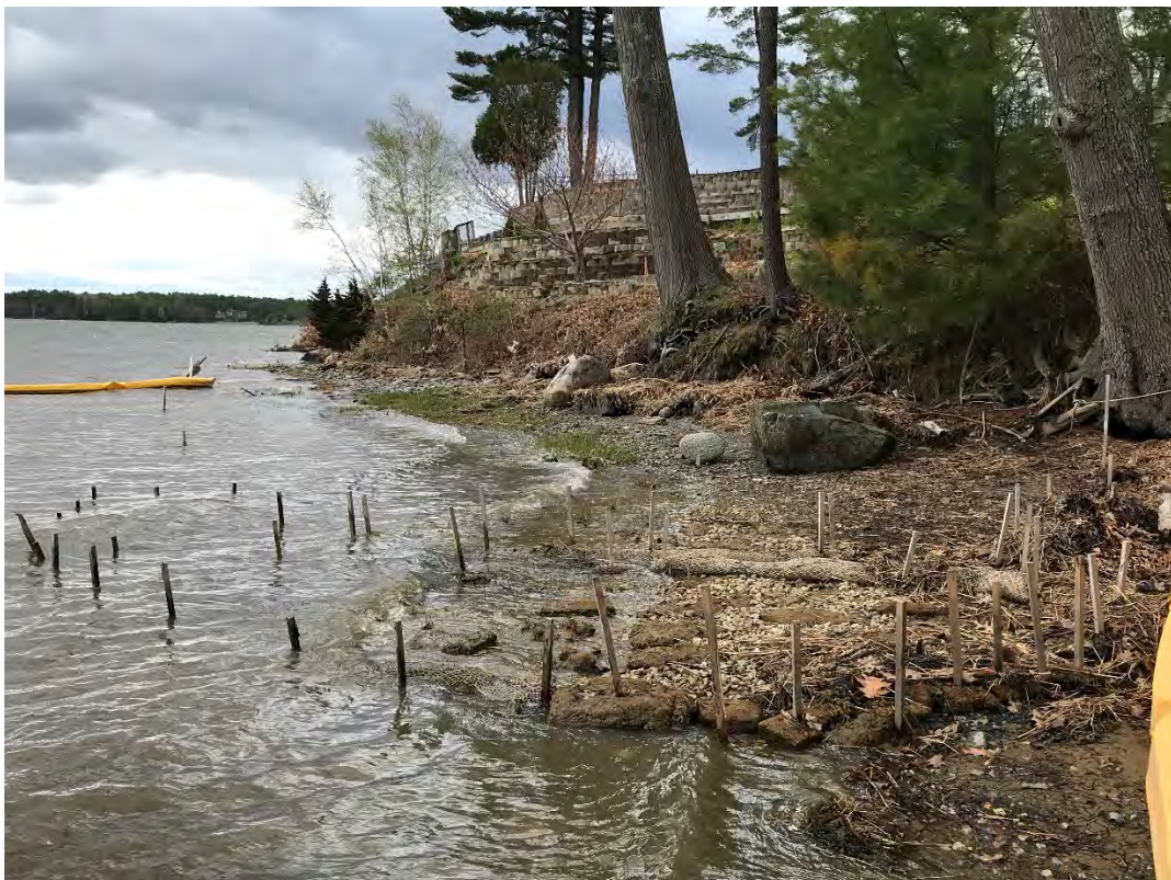
Fig 12: Salt marsh restoration at Gundalow Landing/east side of the bay. Viewing south. (04-30-21)
