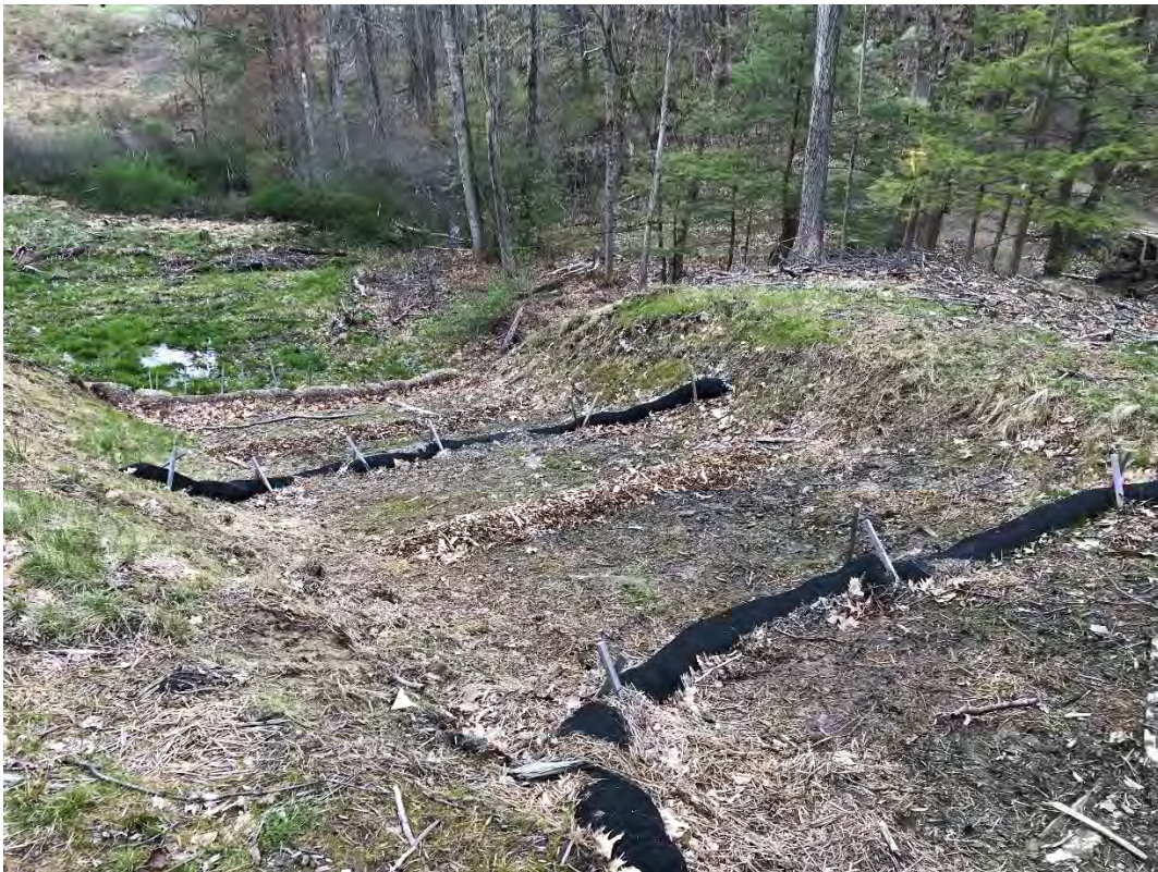
Fig 8: Lower portion of slope between Strs. 28 and 29. Viewing northeast. (04-30-21)
