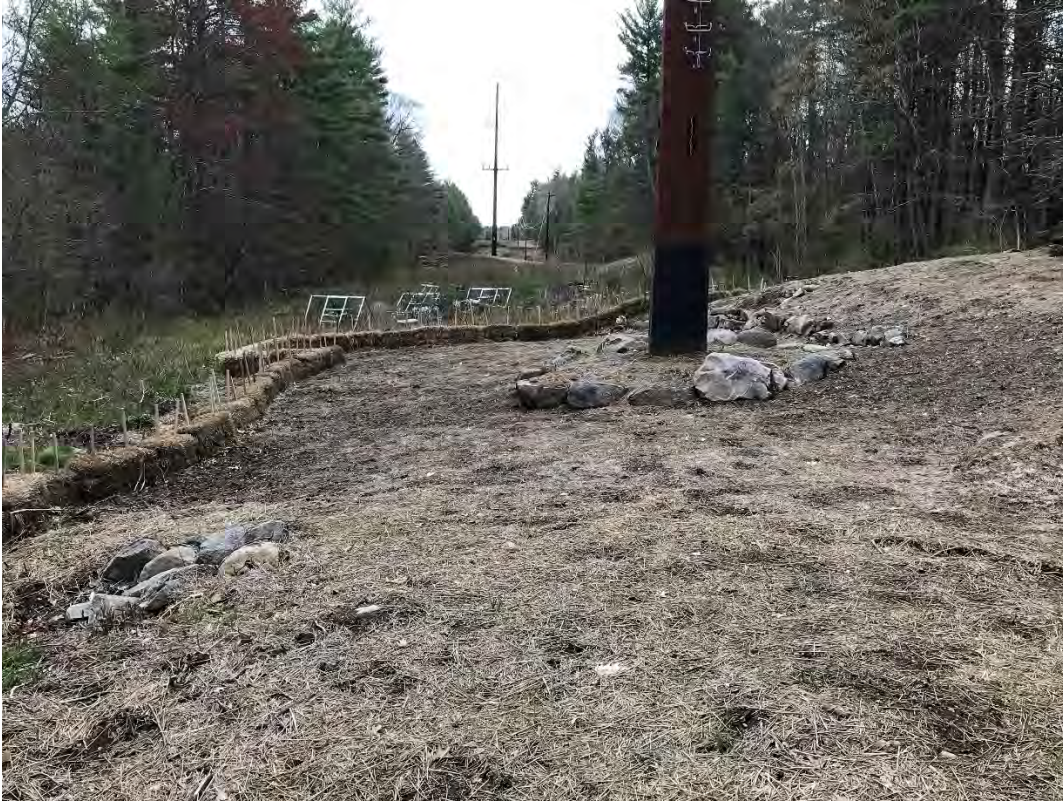
Fig 5: Str. 89 work area. Viewing southeast. (04-30-21)
